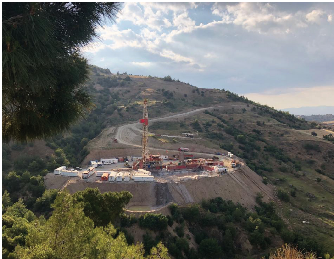
Figure 16. Geothermal drilling in mountainous and remote regions, Alaşehir Türkiye, taken in 2021.
